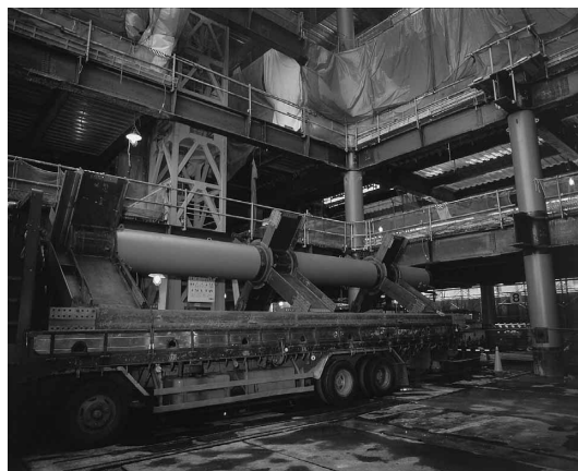
Photo 1 Circular steel column with exterior diaphragm ring “KS Column”
