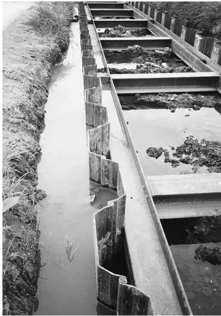
Photo 9 Wide flange steel sheet pile
