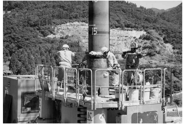
Photo 10 High-strength landslide control steel pipe pile "K-60" with screw joint "Meka-Neji"
