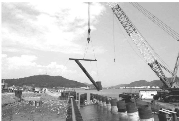
Photo 8 Struttet frame quay-wall structure
