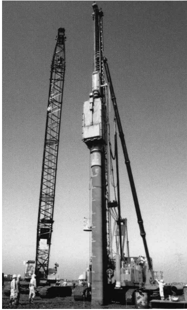
Photo 12 Inner pile excavation method (KING method)
