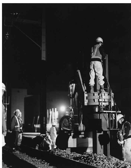
Photo 6 H-shaped steel sheet pile (K-domeru)
