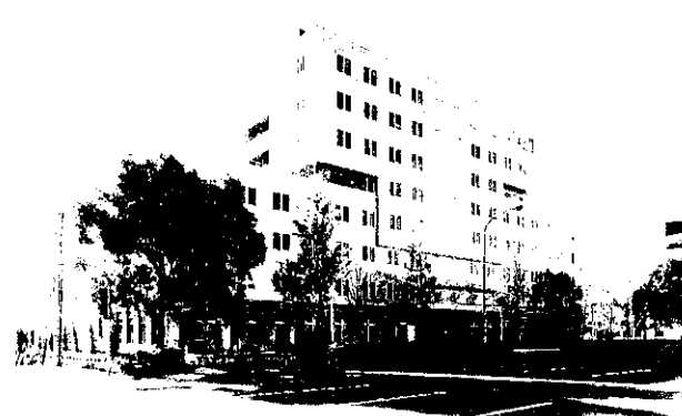
Photo 1 Kobe Head Office Building
