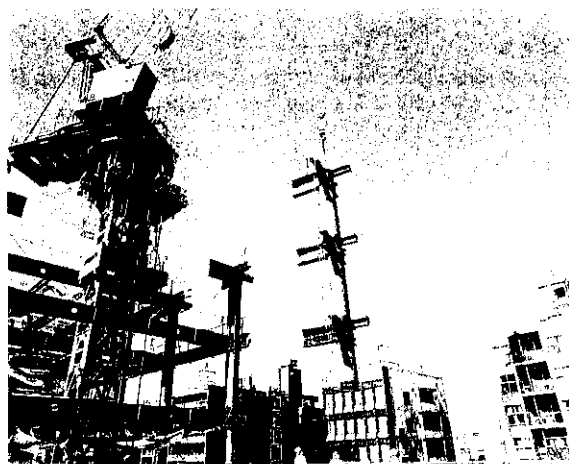
Photo 10 Installation of KS-Column
