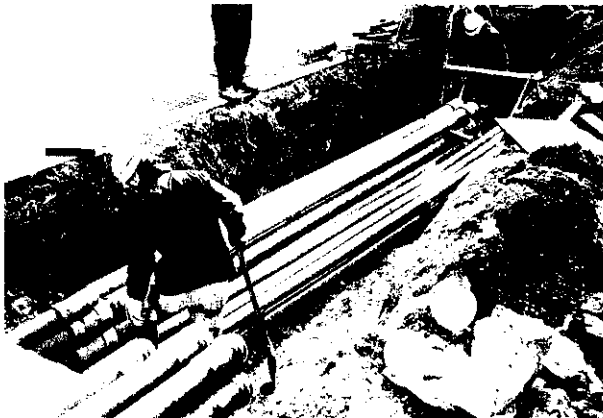
Photo 4 Communication cable box
