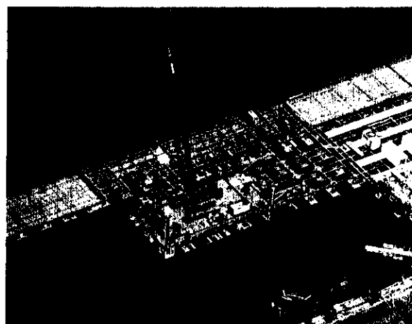
Photo 2 Construction of super platform structure over flood-regulating pond using wagon method
