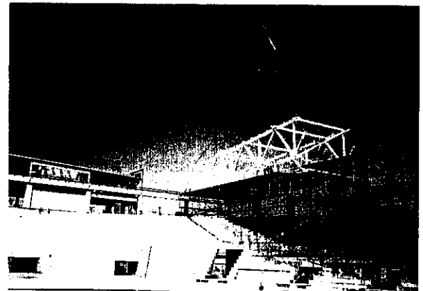
Photo 3 Hoisting boxed truss
