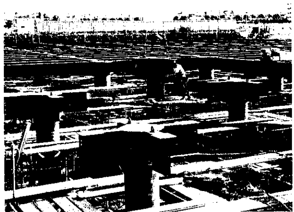
Photo 5 Installation of pile heads by ordinary method
