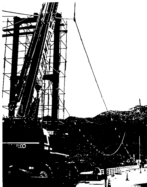
Photo 1 Erection of main cable
