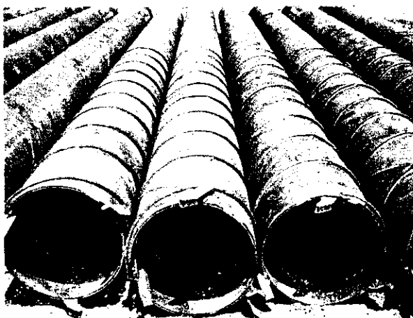
Photo 1 View of drill piles
