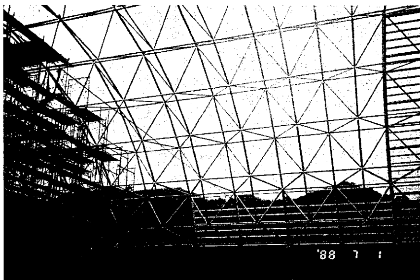
Photo 1 Construction of hall by sliding technique
