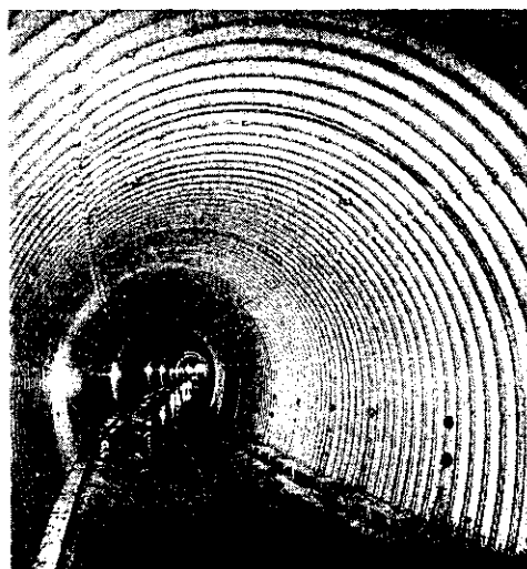
Photo 4 Completed corrugated section with single-side-screw bolts and nuts
