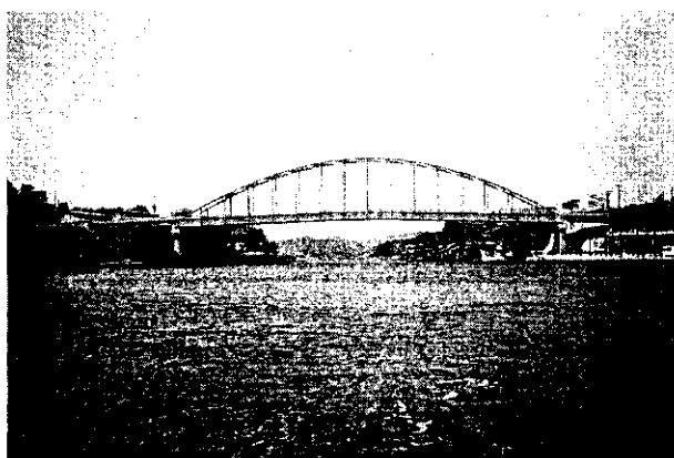
Photo 1 View of Oku-Nagashima bridge
