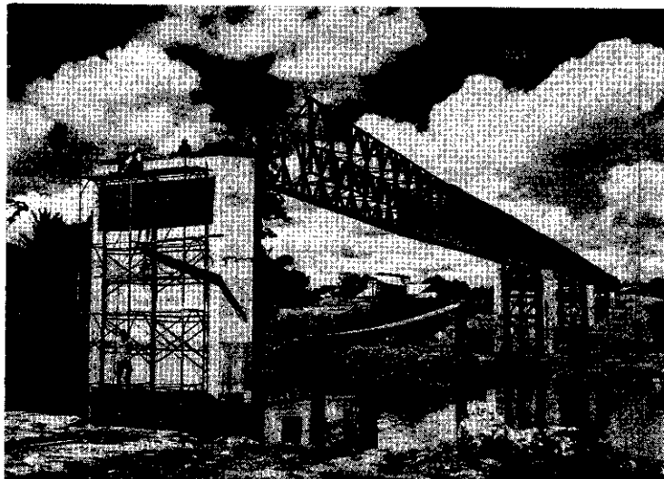
Photo 2 Cantilever launching
