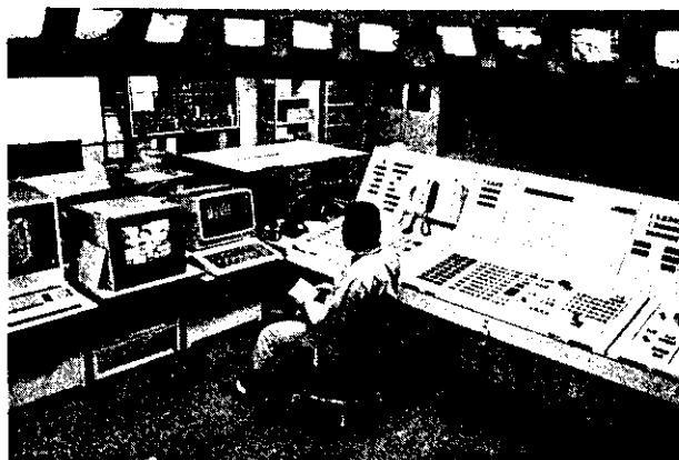
Photo 1 View of yard control pulpit
