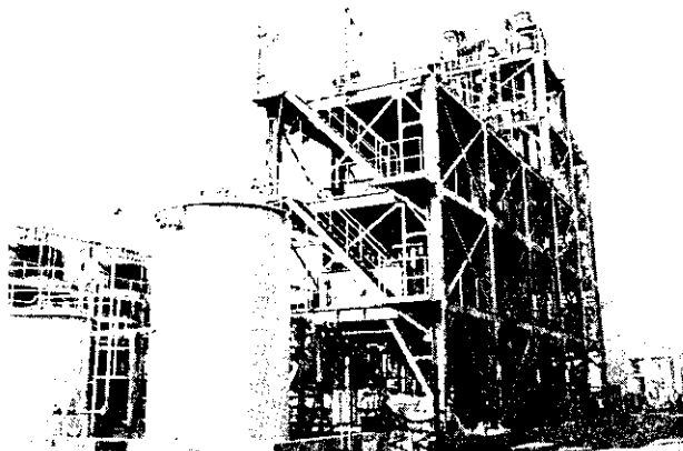
Photo 2 General view of acid recovery plant
