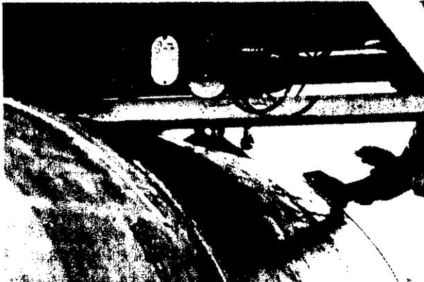
Photo. 3 Circumferential welding of large diameter pipes
