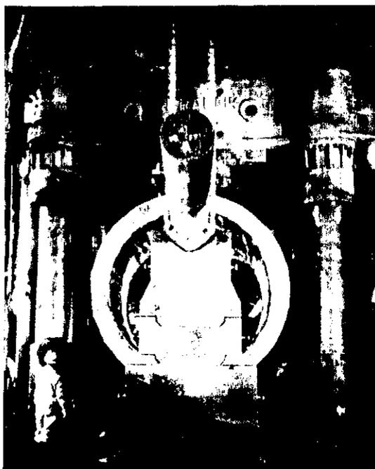
Photo. 5 Forging of shell ring by 6000t press
