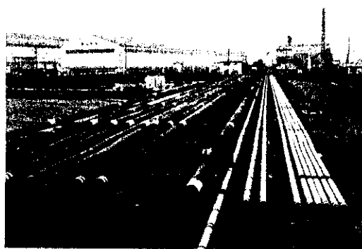
Photo. 3 Prefabrication yard for long pipe
