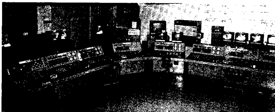
Photo. 3 General view of operation room
