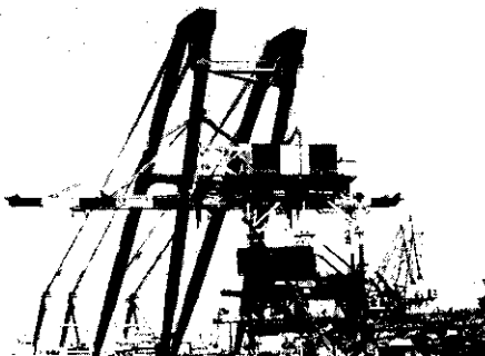
Photo. 2 Fabrication of unloader's upper block by floating crane
