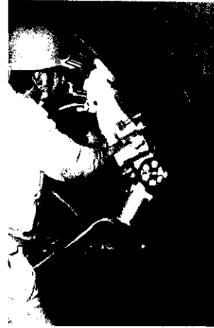
Photo. 13 Welder on the job and welding head
