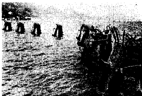
Photo. 2 View of piles driven by diesel pile hammer, Lake Biwa. Angle connectors are used at the top of them
