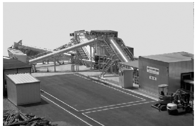
Photo 1 Test plant for wood chip blast furnace feeding
