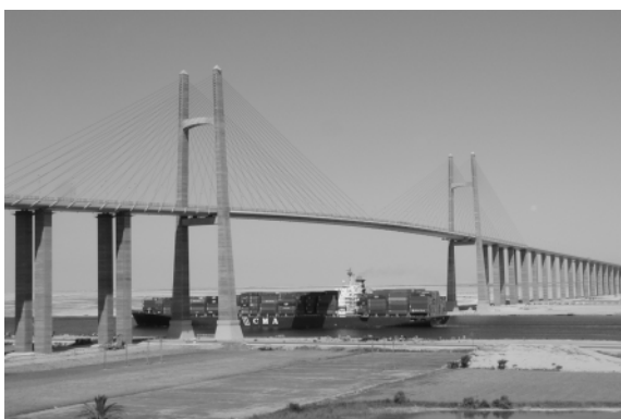
Photo 1 Suez Canal Bridge in Egypt (2001)
