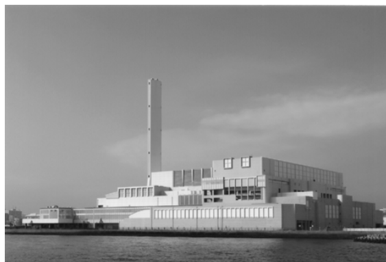
Photo 1 Kanazawa Waste Incineration Plant in Yokohama City
