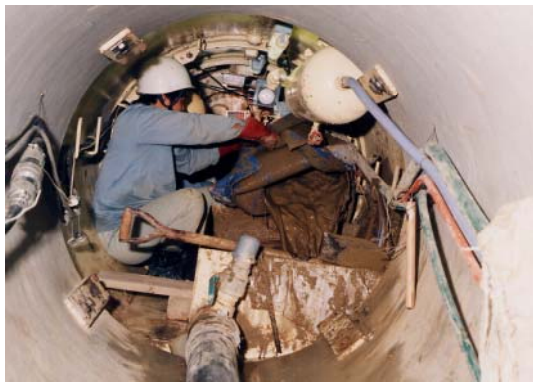
Photo 1 Chamber-man at work
