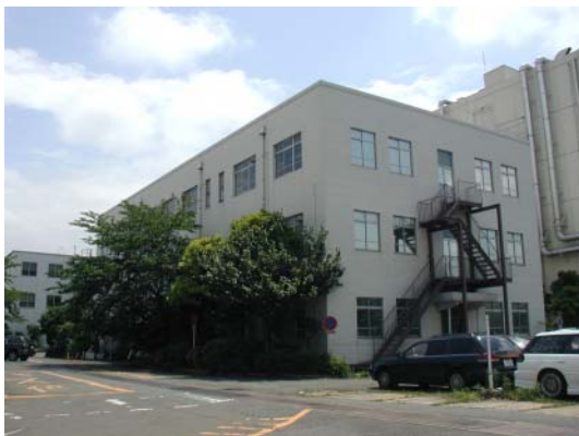
Photo 1 Former Technical Research Department Building (currently NKK Tubes Office)
