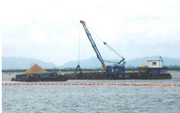
Photo 1 Construction of sand-capping with BF slag sand in Naka-umi, Shimane Prefecture
