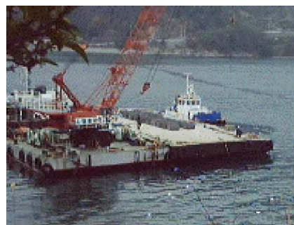
Photo 7 Construction scene for marine environment improvement tests in Hiroshima Prefecture
