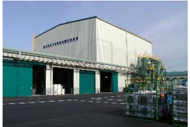
Photo 1 Overall view of the facilities
