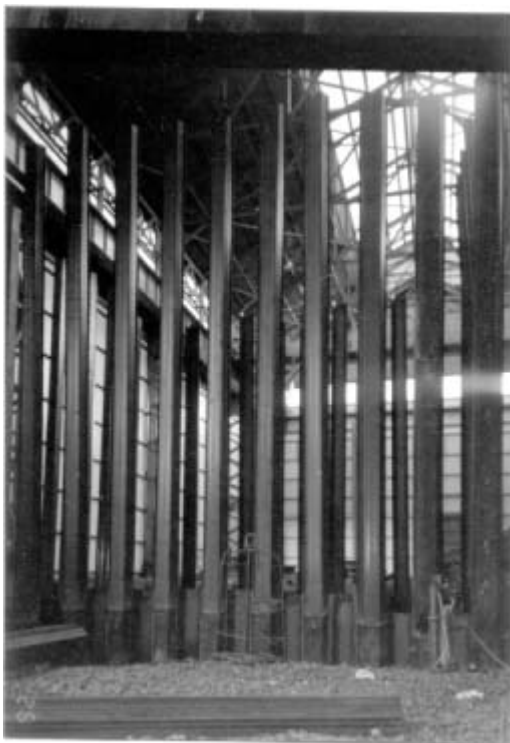
Photo 2 Steel pile jointing
