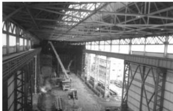
Photo 1 Steel pile driving
