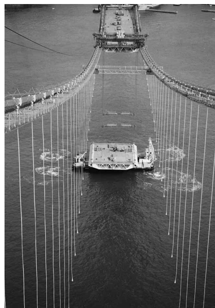
Photo 3 Execution by the direct hoisting method
