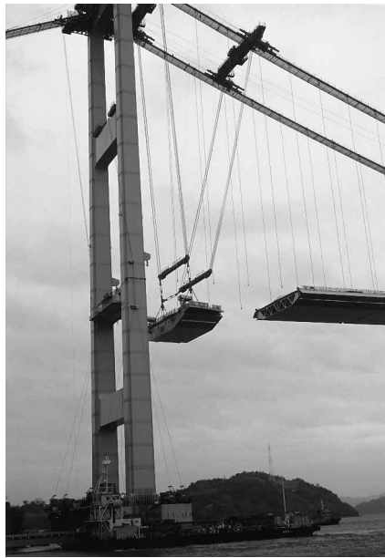
Photo 4 Stiffening girder under the swing erection
