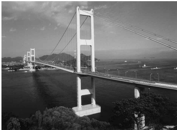
Photo 1 View of 3rd Kurushima Kaikyo Bridge
