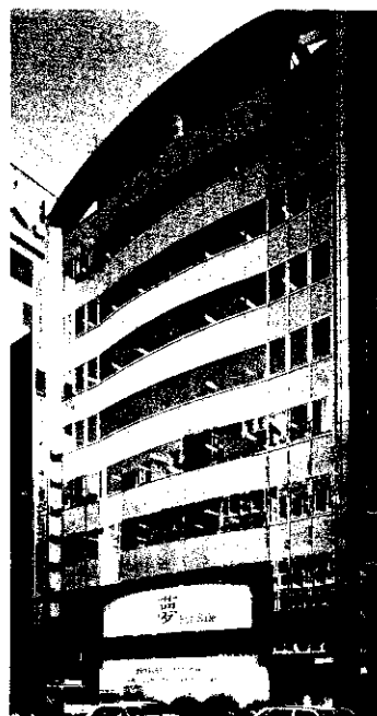
Photo 2 Application of River Wall Metallic to outer walls for buildings (Ginza Iwasaki Building)
