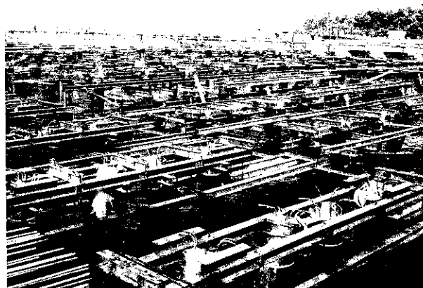
Photo 2 Support system for superstructure
