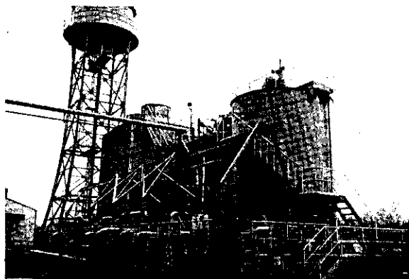
Photo. 3 General view of recirculating water facility
