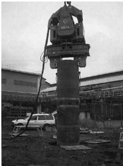
Photo 2 Vibro method test (Used protection cap)
