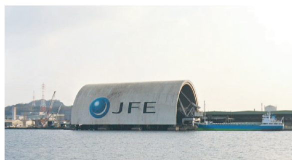
Photo 1 All-weather type (rainy weather cargo handling) shipping berth
