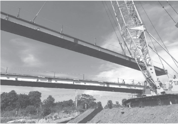
Photo 1 Girder erection by crane (Lao P.D.R)
