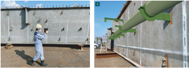
Fig. 13 Checking scene of installation position of drainage fittings
