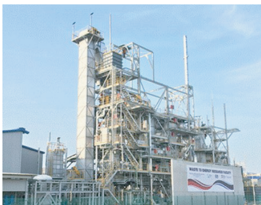
Photo 2 High-temperature gasifying and direct melting furnace demonstration facility
