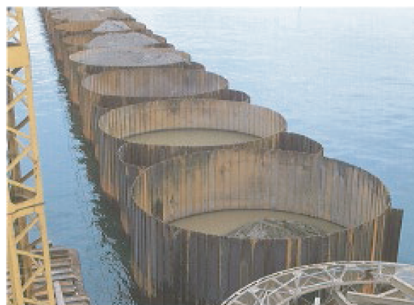
Fig. 2 Steel sheet pile cell method
