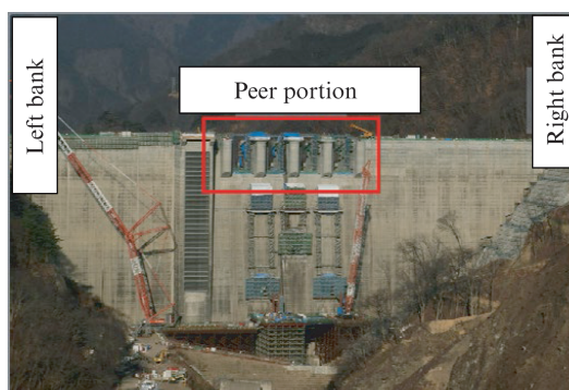
Photo 4 Installation position of sluice gate
