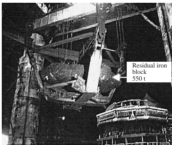
Photo 3 Hanging up large residual iron block
