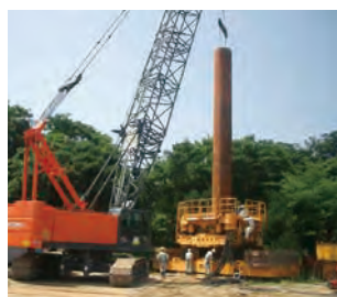
Toe wings and a construction method of the JFE Tsubasa Pile™
