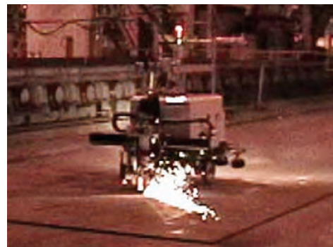
Automation of steel plate conditioning work
