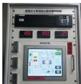
High pressure hydrogen gas permeation test device (1000bar)
