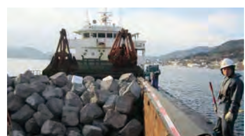
Artificial stones used in disaster recovery in Tohoku area (1 ton size)
