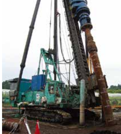
Pile head rotation type (Batter pile)
