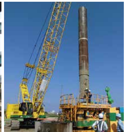
Piler set over a main pile
