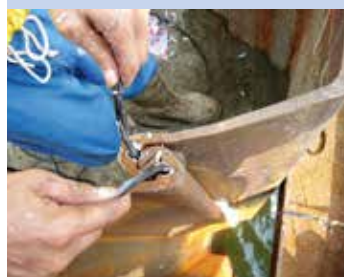
Injection of filler material (silicone)
