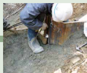
● Check of filling condition
