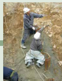
● Pulling out of pre-stressed concrete steel wires
