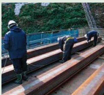
● Installation of sealing rubber along pockets
