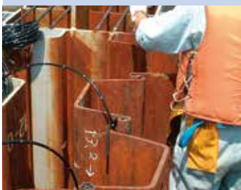
Insertion of filler injection tube
