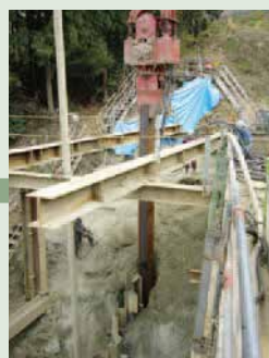
● Piling by vibratory hammer
