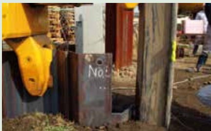
● Execution at a corner overlapping area
