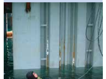
Checking of filling condition by divers
