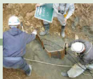
● Injection of filler material (silicone)
