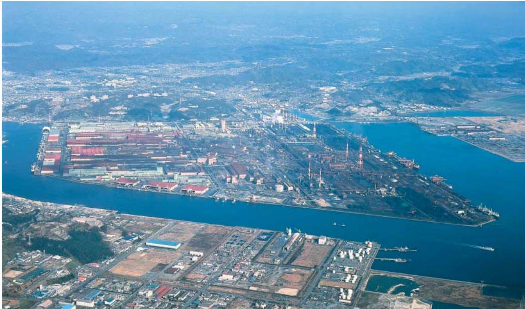
◀ West Japan Works (Fukuyama)
