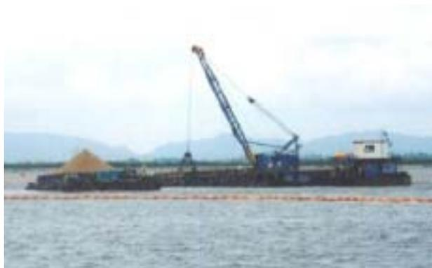
Photo 1 Construction of sand capping with granulated blast furnace slag in Nakaumi, Shimane
