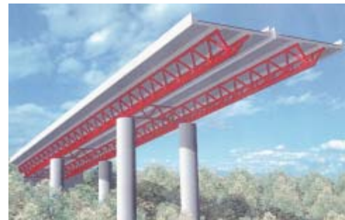
Fig.1 Image of a pipe-truss bridge
